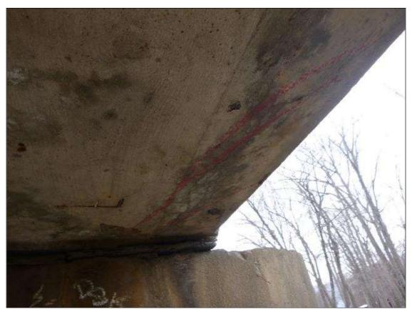
Span 1 Beam 3: BOTTOM OF BEAM AT PIER 1, DELAMINATION 18 INCHES LONG BY 6 INCHES WIDE
