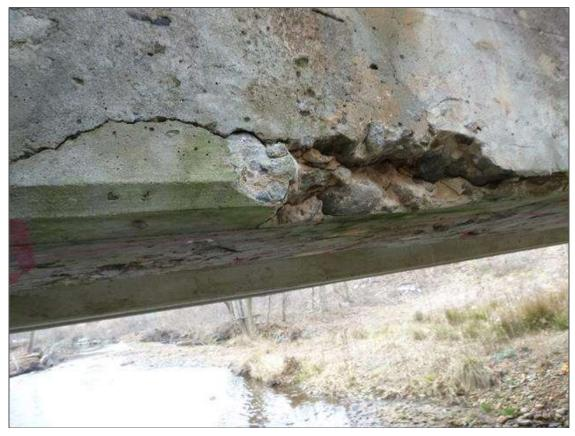
Span 2 Beam 1: 9 FEET FROM END BENT 2, ON BOTTOM AND SOUTH FACE OF BEAM, DELAMINATION 56 INCHES LONG BY 18 INCHES WIDE ON BOTTOM AND 10 INCHES HIGH ON SOUTH FACE
