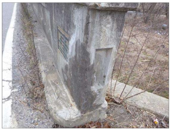
Span 1 Right Bridge Rail: AT WEST END, 3 SQUARE FEET OF UNSOUND PATH WITH EFFLORESCENCE
