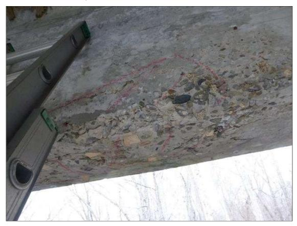
Span 2 Beam 1: 9 FEET FROM END BENT 2, ON BOTTOM AND SOUTH FACE OF BEAM, DELAMINATION 56 INCHES LONG BY 12 INCHES WIDE ON BOTTOM AND 10 INCHES HIGH ON SOUTH FACE
