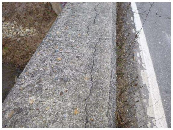
Span 2 Left Bridge Rail: LONGITUDINAL CRACKING TO FULL LENGTH OF TOP OF RAIL
