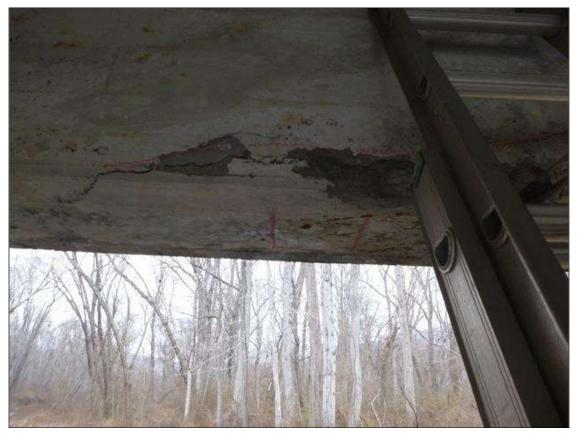
Span 2 Beam 1: 9 FEET FROM END BENT 2, ON BOTTOM AND SOUTH FACE OF BEAM, DELAMINATION 56 INCHES LONG BY 12 INCHES WIDE ON BOTTOM AND 10 INCHES HIGH ON SOUTH FACE
