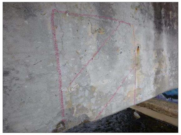
Span 2 Beam 3: 18 FEET FROM BENT 1, DELAMINATION ON RIGHT FACE OF BEAM 18 INCHES LONG BY 18 INCHES HIGH
