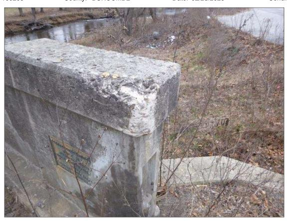
Span 1 Right Bridge Rail: 10 INCHES LONG X 6 INCHES HIGH X 1 INCH DEEP SPALL IN TOP OF RAIL AT ABUTMENT 1
