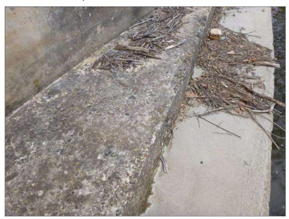
End Bent 2 Abutment: HEAVY SCALING/SPALLING (22 FEET X 1 FEET X 4 INCHES) IN FOOTING APRON AT DOWNSTREAM END
