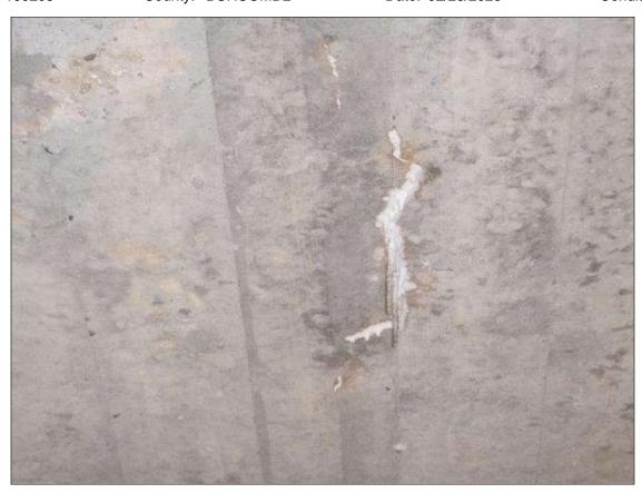
Span 1 Deck: 12 INCHES OF EFFLORESCENCE BUILDUP IN BOTTOM OF DECK, MIDSPAN BAY 1
