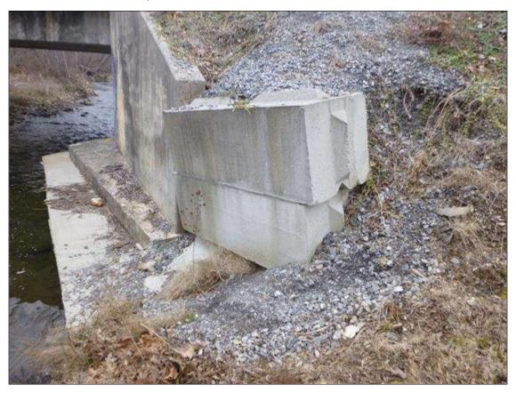
CONCRETE WINGWALL AT SOUTHEAST CORNER IS ROTATED TOWARD THE STREAM.
