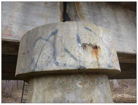
Bent 1 Cap 1: MAP AND VERTICAL HAIRLINE CRACKING TO RIGHT END OF CAP
