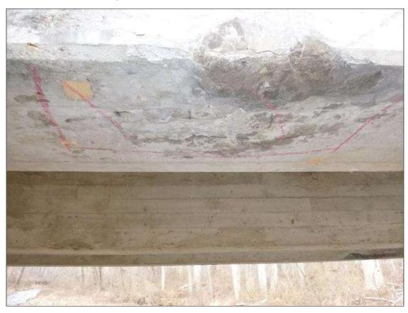
Span 2 Beam 3: 17 FEET FROM BENT 1, UNSOUND PATCH ON BOTTOM OF BEAM, 2 FEET LONG BY 1 FOOT WIDE
