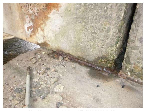
Span 2 Beam 1 - Near Bearing 1: SURFACE CORROSION
