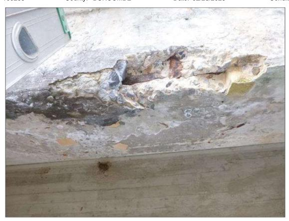
Span 2 Beam 3: (PROMPT ACTION REQUEST) 23 FEET FROM BENT 1, BOTTOM RIGHT CORNER OF BEAM, SPALL WITH EXPOSED MAIN REINFORCING 3 FEET LONG BY 9 INCHES WIDE BY 2 INCHES DEEP
