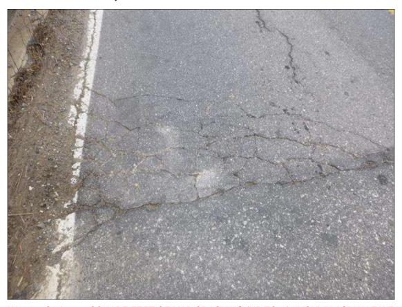
Span 1 Wearing Surface: 5 SQUARE FEET OF MAP CRACKING (UP TO 1/4 INCH) IN ASPHALT WEARING SURFACE AT NEAR LEFT SIDE. 3 SQUARE FEET OF MAP CRACKING (UP TO 1/4 INCH) IN ASPHALT WEARING SURFACE AT NEAR RIGHT SIDE.
