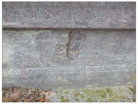
Span 2 Right Bridge Rail: (6) SPALLING WITH EXPOSED REBAR THROUGHOUT INSIDE SIDE OF PARAPET (UP TO 10 INCHES X 6 INCHES X 3/4 INCH)
