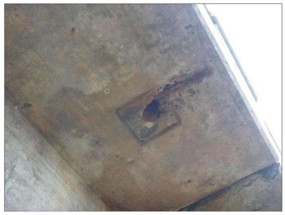
Span 1 Deck: SPALL (10 INCHES X 6 INCHES X 1 INCH) WITH EXPOSED REBAR WITH SECTION LOSS AT FAR RIGHT DECK OVERHANG 2 FEET FROM PIER 1
