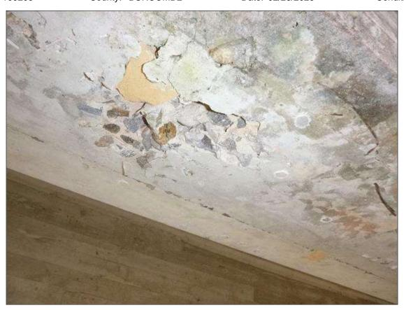
Span 2 Beam 1: 21 FEET FROM BENT 1, BOTTOM OF BEAM, 9 INCH DIAMETER BY 1/2 INCH DEEP SPALL
