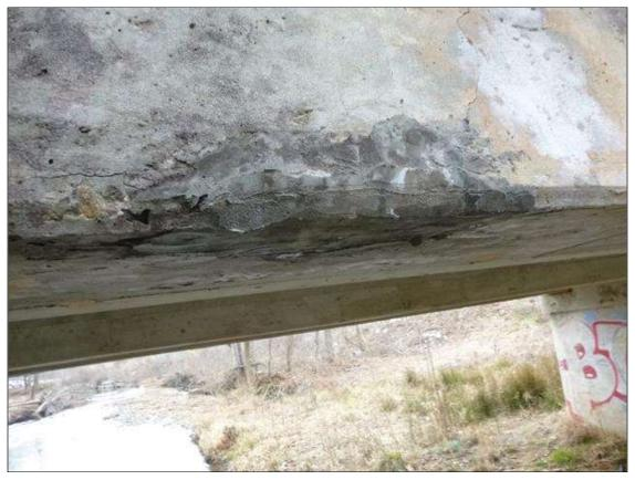
Span 2 Beam 1: SOUND PATCH AT MIDSPAN, BOTTOM LEFT OF BEAM 12 INCHES BY 6 INCHES
