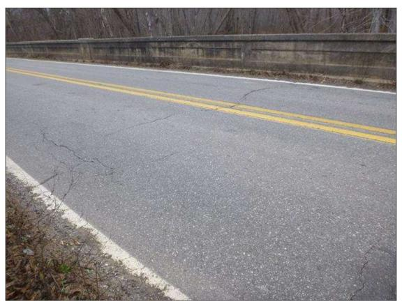
Span 2 Wearing Surface: INTERMITTENT TRANSVERSE, LONGITUDINAL AND MAP CRACKING (UP TO 1/2 INCH)
