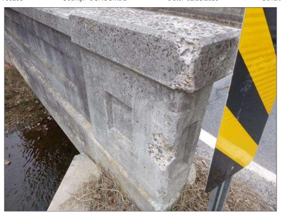
Span 2 Right Bridge Rail: AT END OF RAIL, (2) SPALLS UP TO 7 INCH DIAMETER BY 1/2 INCH DEEP
